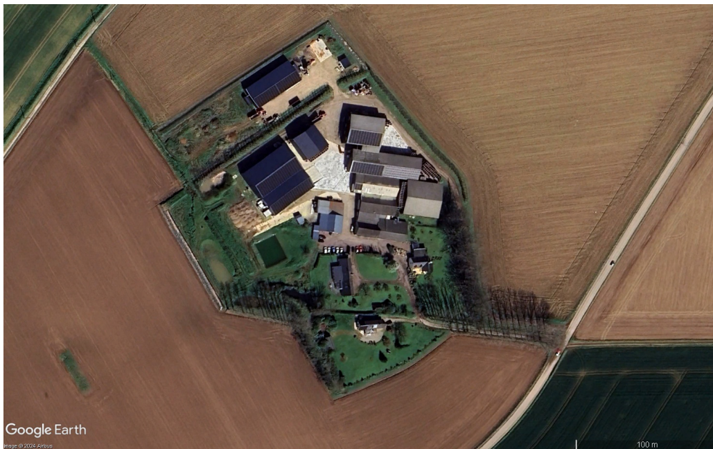
Clos-masure being filled in by sheds.
